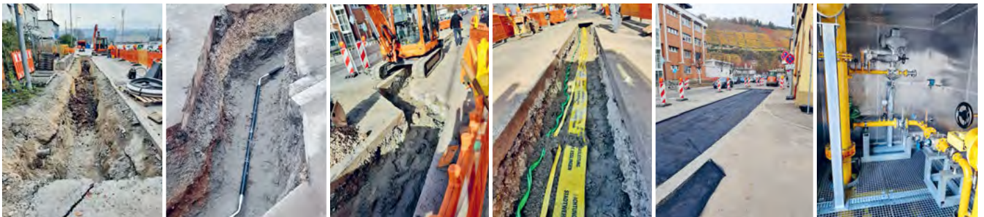
Road closure and trench excavation
