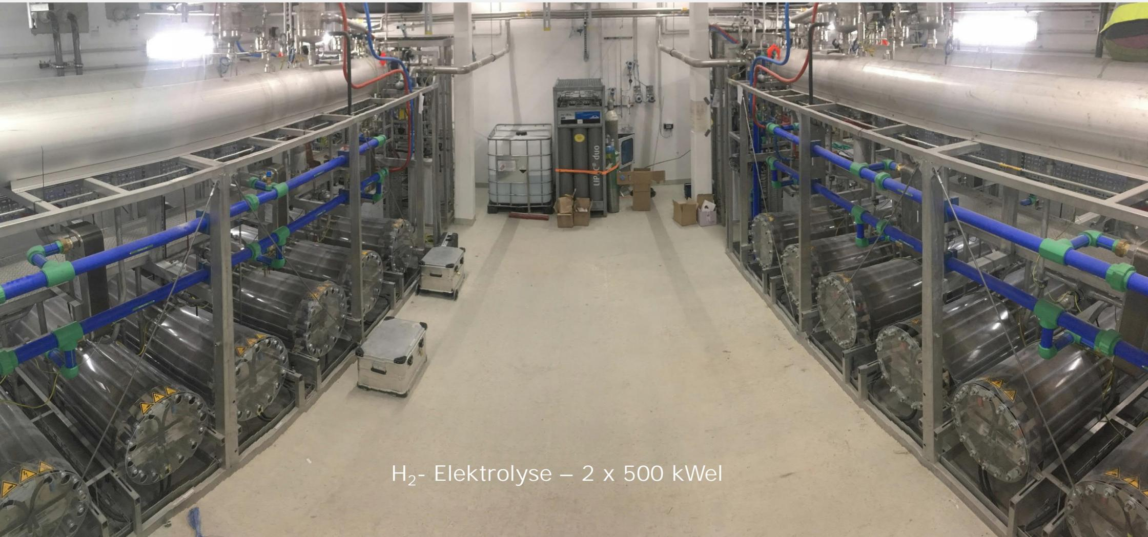
H<sub>2</sub>- Elektrolyse – 2 x 500 kWel
